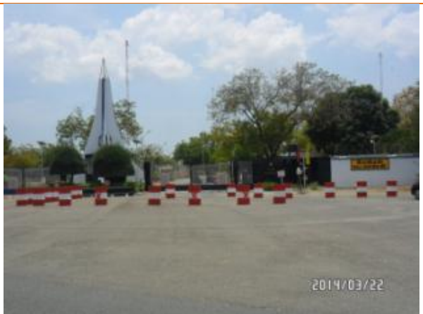
INS Kottabomman , Boundary wall along SH89 on RHS from Km 12/600 to Km 16/00
