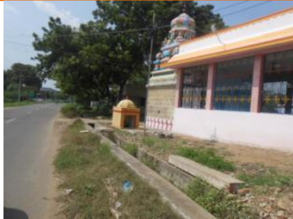
Road side structure
