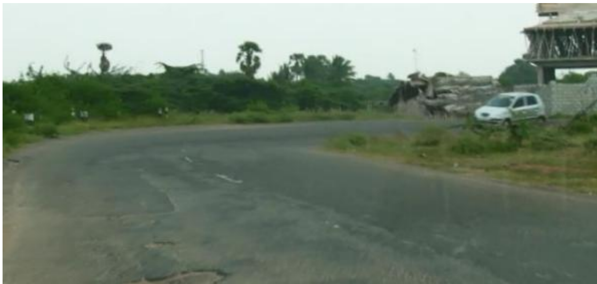
Sharp Curve (1) at Chainage 26+440, SH89
