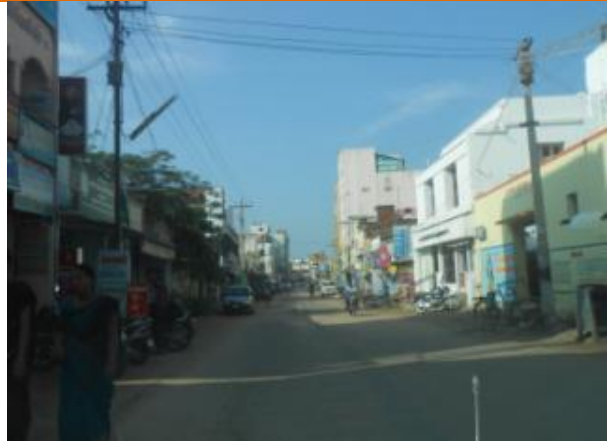
Market Area At km 43.400
