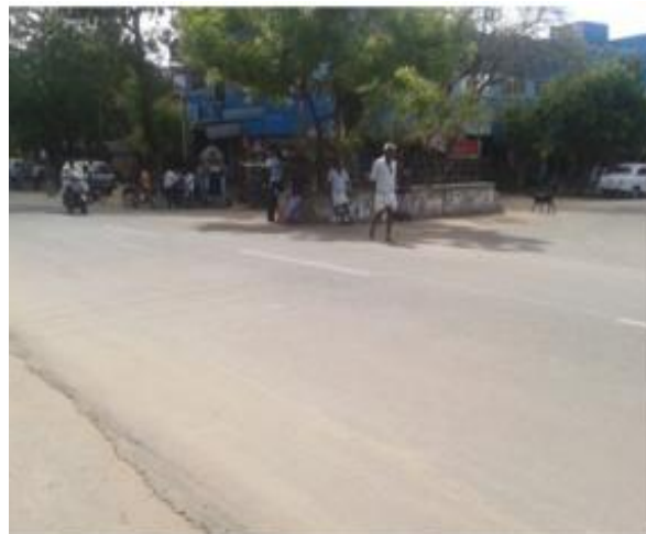
End Point at Ch. 35+800
