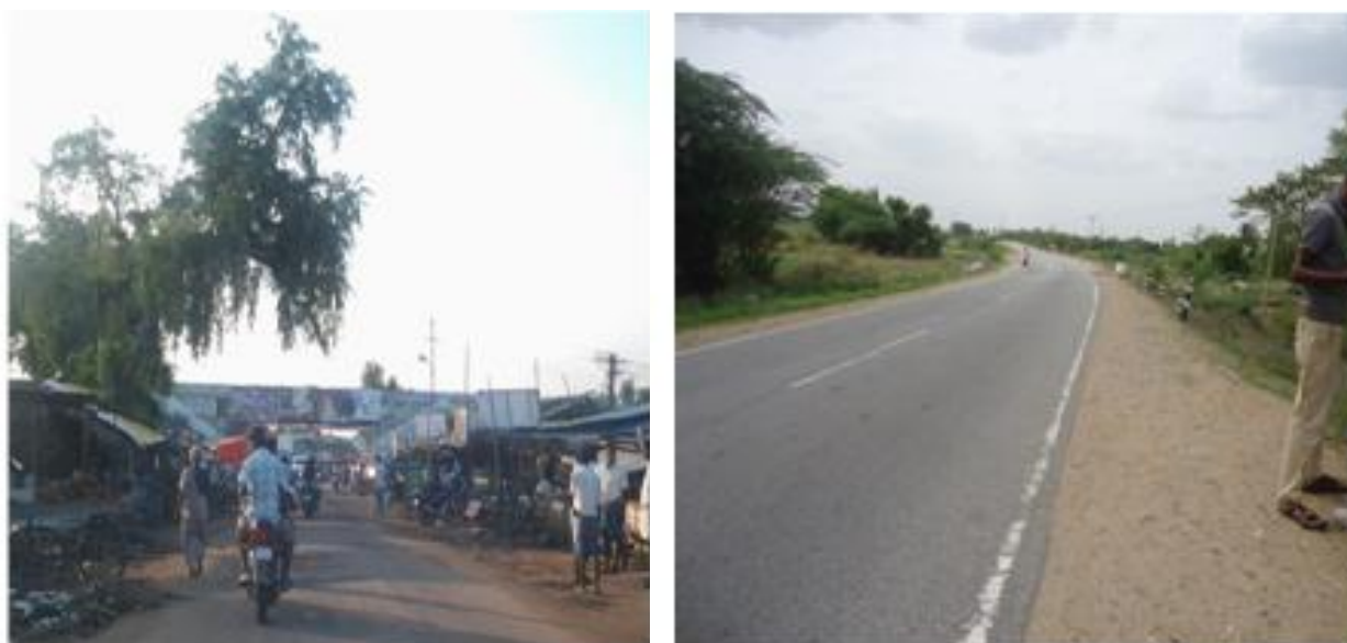
Start Point at 41+700 near Madapattu End Point (Proposed Jn. of SH-9 with SH-137)
