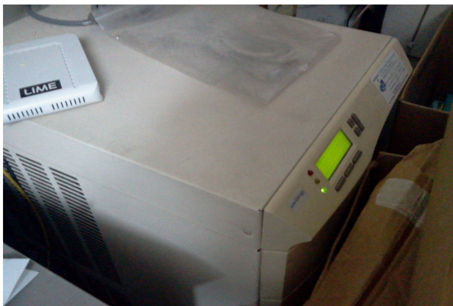
Figure 2.7: St. Ann's Bay's UPS
