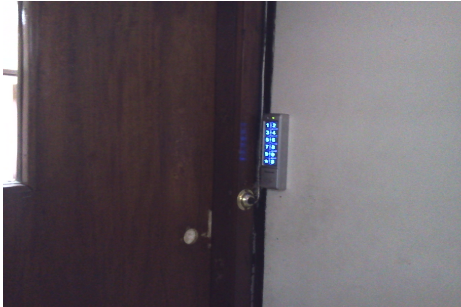
Figure 2.2: Server room entry with keypad
