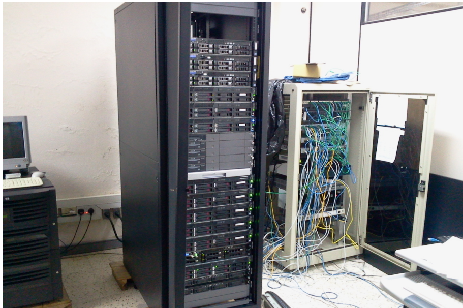
Figure 2.3: 3rd Floor cable distribution and 18KVA UPS
