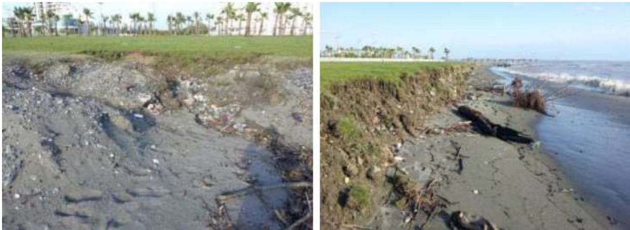
Figure 6-28 – Sediment Erosion along the Shoreline at Anaklia (Source: DOWHA Engineering Co, 2011).
