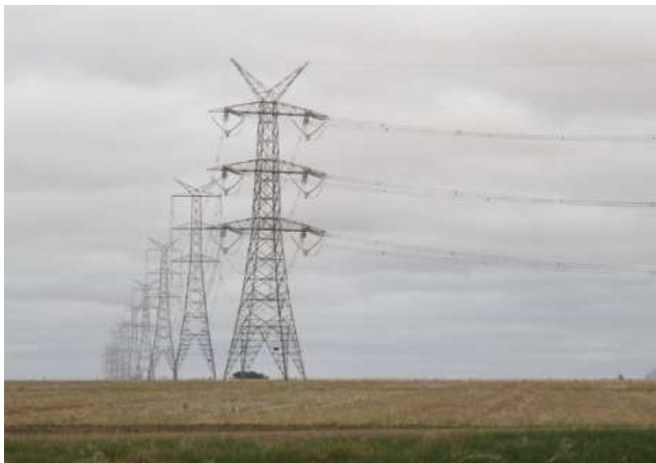
Figure 2-11 – Example of a standard 500 kV OHL
