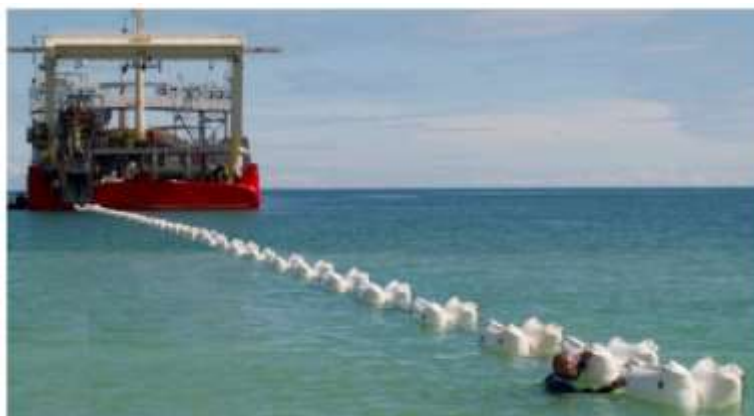
Figure 2-15 – Submarine cable landing operation.
