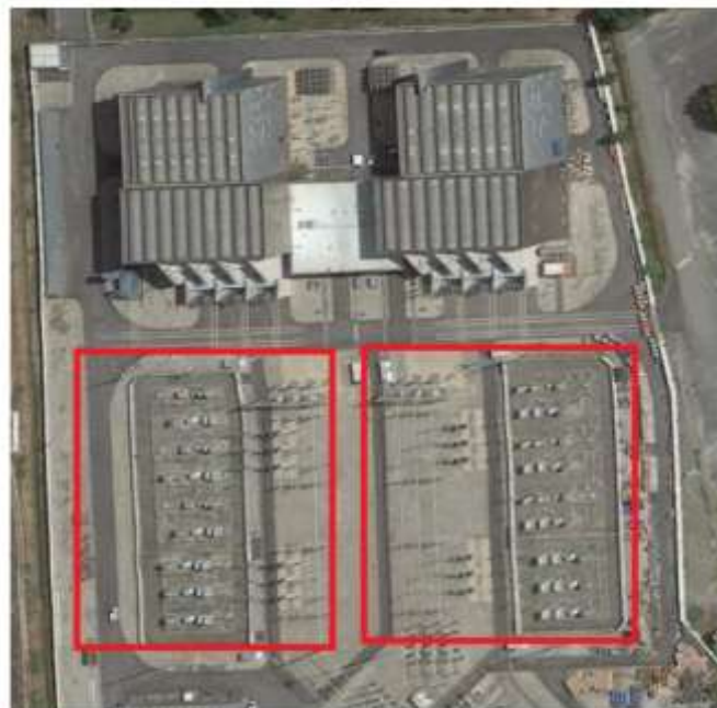
Figure 5-10 – Footprint of a 1000 MW bipolar LCC converter station (Latina converter station of SAPEI Interconnector). OThe overall footprint is 48,000 sqm; the area occupied by the AC filters is marked in red.
