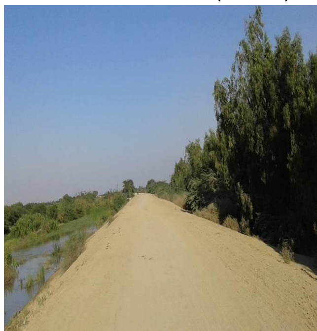
Picture 4: View of Indo Bund (End Point)
