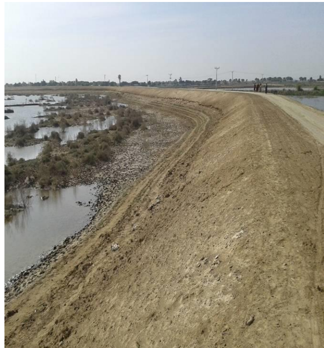
Picture 4: View of wind eroded area of BU bund
