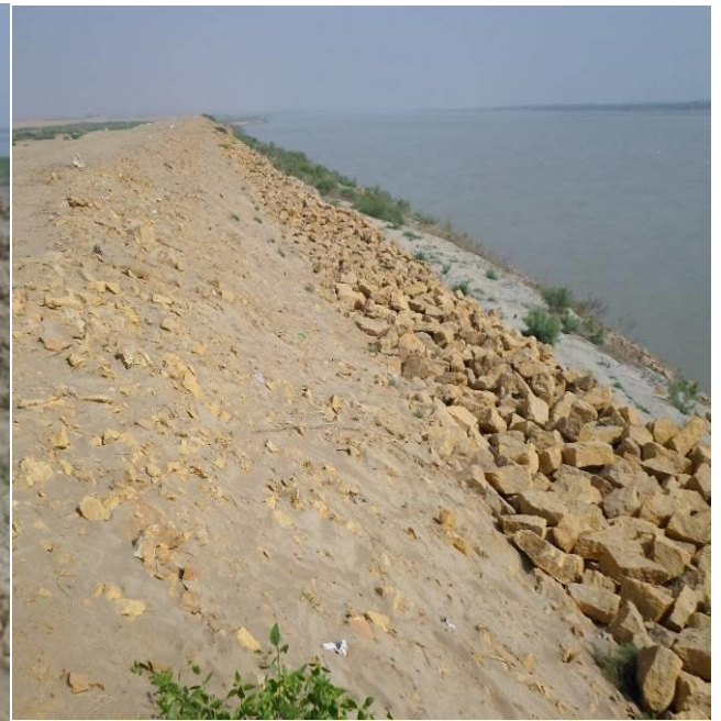
Picture 2: View of SH bund (River Side)
