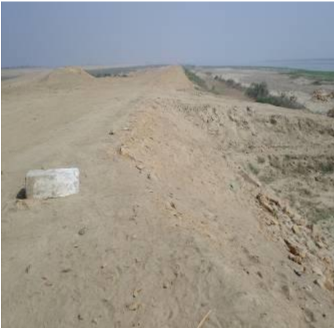
Picture 1: View of SH bund
