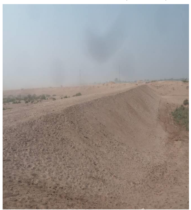
Picture 4: View of SH bund (start point)
