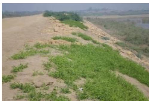
Jaar observed at embankment of BU Bund
