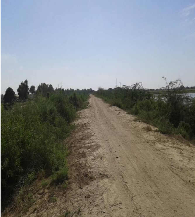
Picture 1: View of MS bund
