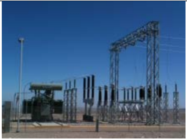
2. Electrical substation next to the solar panels
