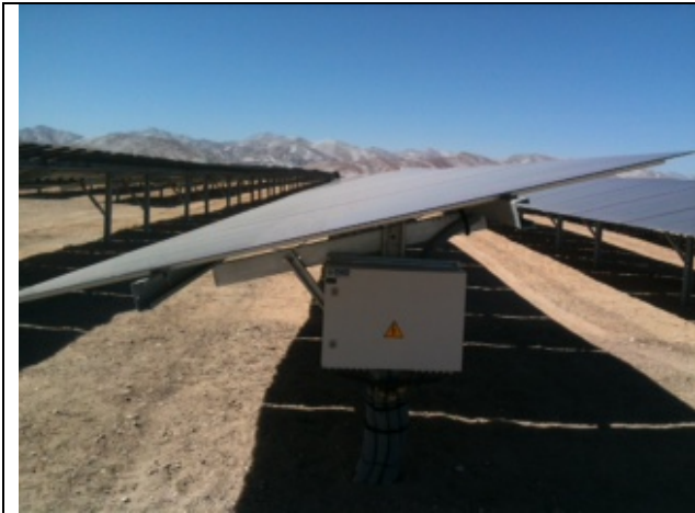
1. Solar panel arrays
