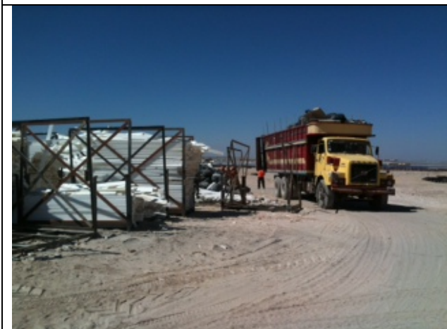
5. Disposal of recyclable and reusable materials
