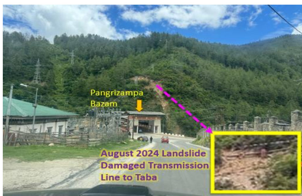
Figure 3: Climate vulnerability of LRCP components highlighted by the August 2024 Dechencholing flood. A short, intense rainfall event triggered both a landslide damaging the raw water transmission line and a flash flood that damaged the Bus Priority Service Road.
