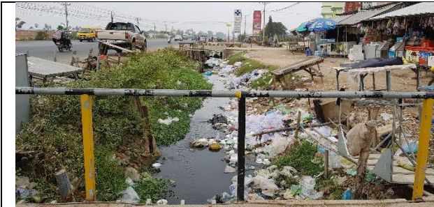
PK22+000, Solid waste on existing drainage
