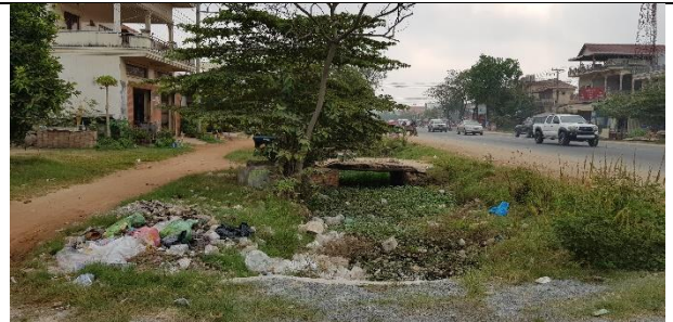
PK22+000, Solid waste on existing drainage
