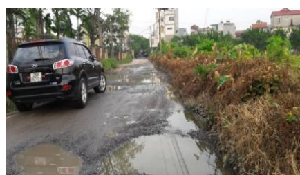
Residential area at lane 56, Ngo Xuan Quang road
