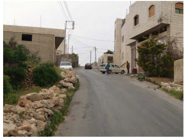
Plate 6: Khalit Addar village: steep slope, residential homes, stone walls, underground (non-municipal) sewer line, cesspits (assumed if not connected to sewer line), aboveground utility lines
