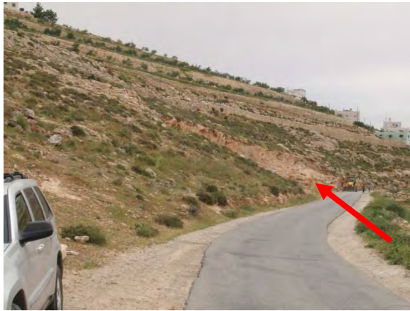
Plate 13: Local road looking towards Khalit Addar and stone quarry (see red arrow and Plate 12)
