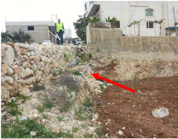
Plate 5: Exposed 2" water pipeline (see red arrow)
