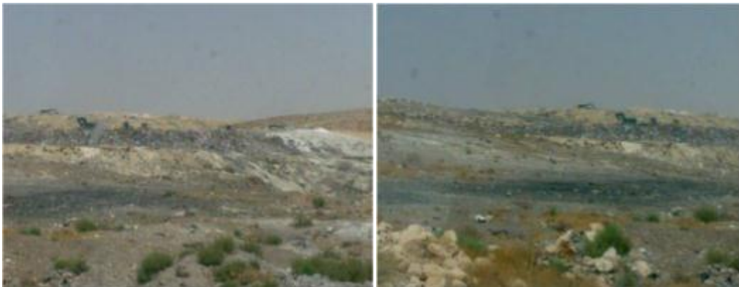
Figure 4.13: Yatta dumpsite receiving SW from Hebron and Bethlehem LGUs
