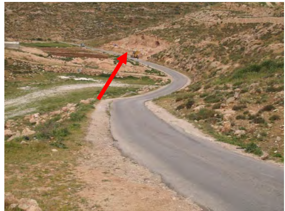
Plate 12: Local road: single-lane paved road, rock-face terrain, open agricultural land, and stone quarry (see red arrow)
