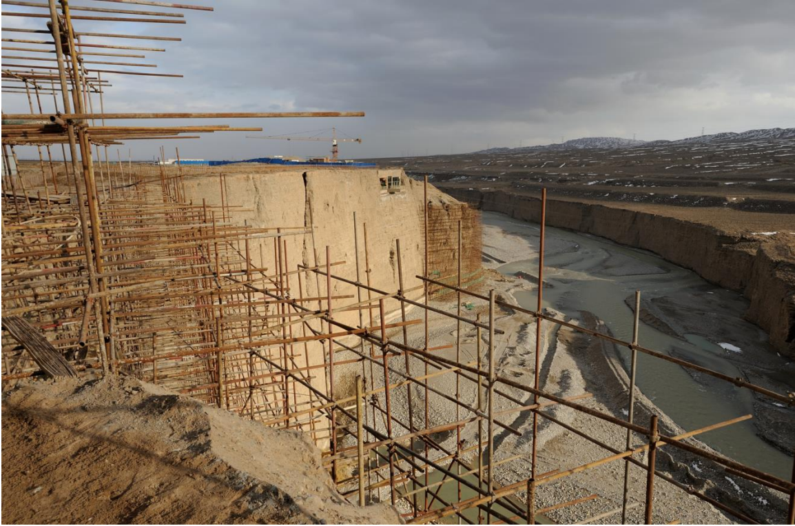
Jiayuguan Conservation and Stabilization Works
