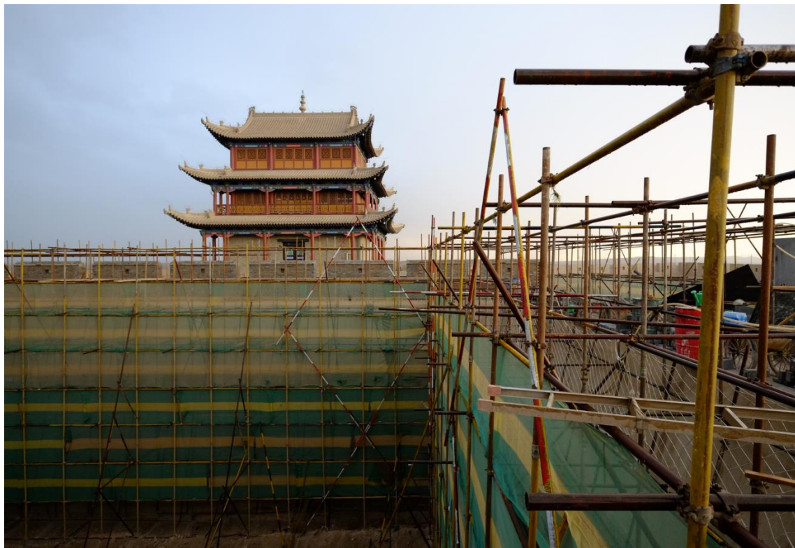
Jiayuguan Great Wall Conservation Works
