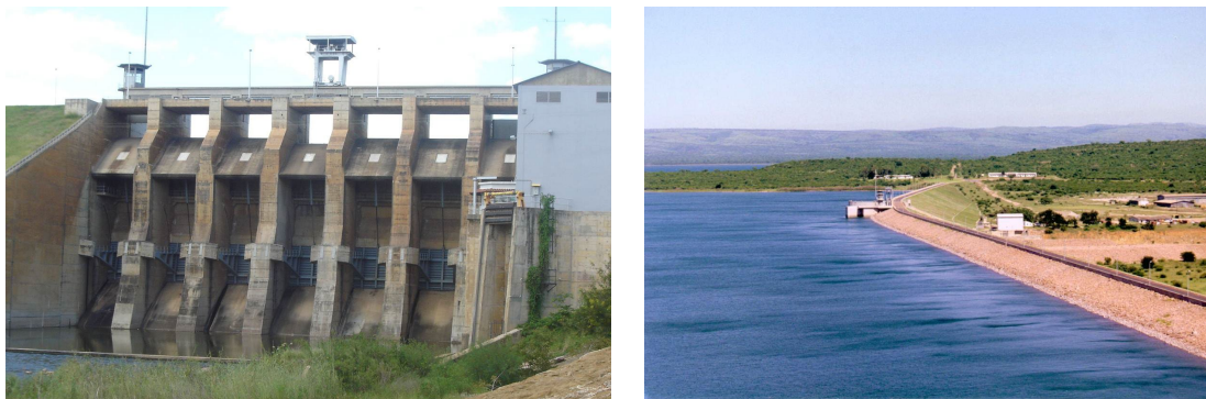
Figure 6-37 – Pequenos Libombos Dam
