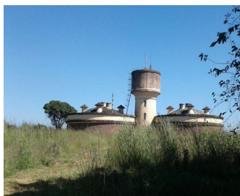
Water tanks, Namaacha
