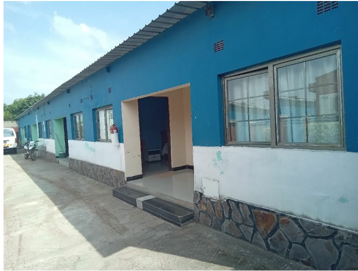
Figure 6-164 – Pérola guesthouse on the Line's RoW
