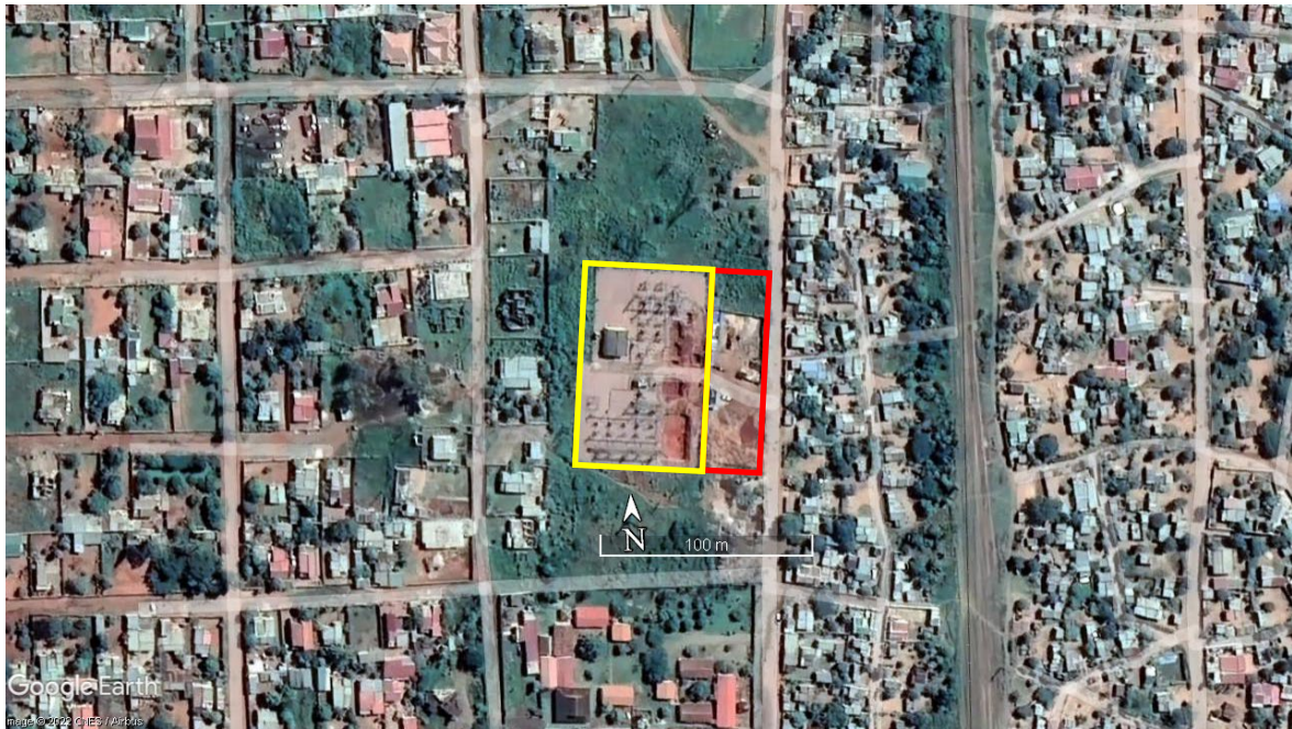
Figure 4-5 – Existing Boane substation (yellow) and proposed extension (red)
