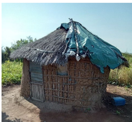
House in Gumbe
