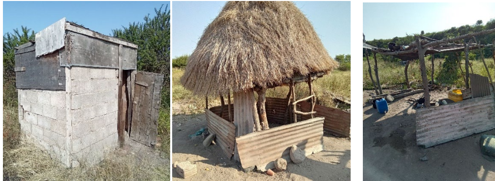
Figure 6-3 – Diverse Selection of Impacted Auxiliary Structures
