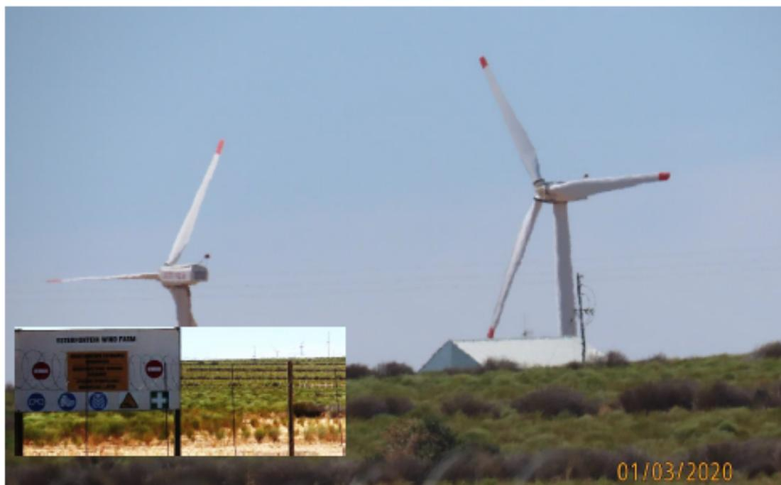
Figure 2: Red-tipped turbine-blades on turbines at the Ysterfontein wind farm north west of Clanwilliam in the Western Cape (S 32° 9'23.42" E 18°49'7.10"). While these mitigations are not used in the correct single-blade configuration used by the Norwegians, they set a precedent for turbine blades to be red-painted in South Africa © RE Simmons
