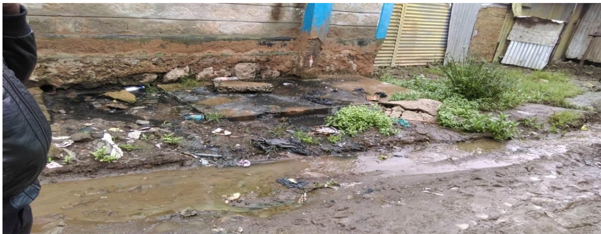
Plate 9: Overflow from a septic tank
