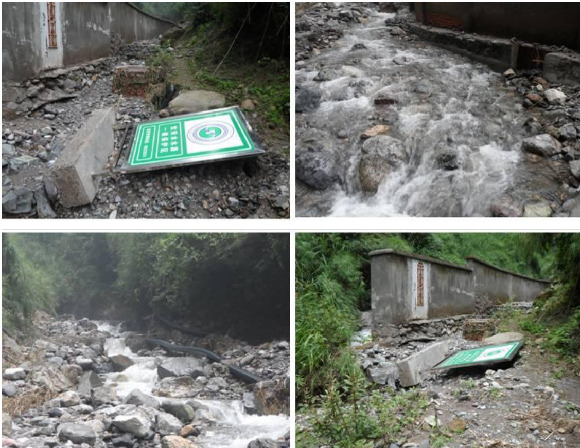
Fig. 2-3 Mountain stream for water supply at Jiaochanggou
