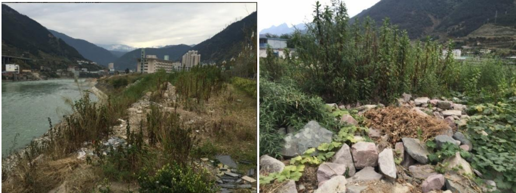
Figure 2-7 Current Situation of Flood Control Embankment in Shimian County
