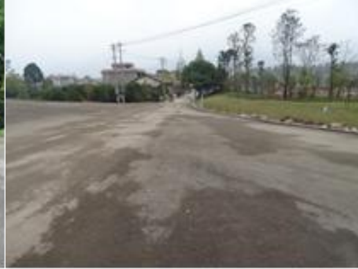
Settlement in Yanwei Village at Z2K0+050~Z2K0+350
