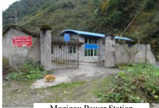
Mozigou Power Station (K28+100)
