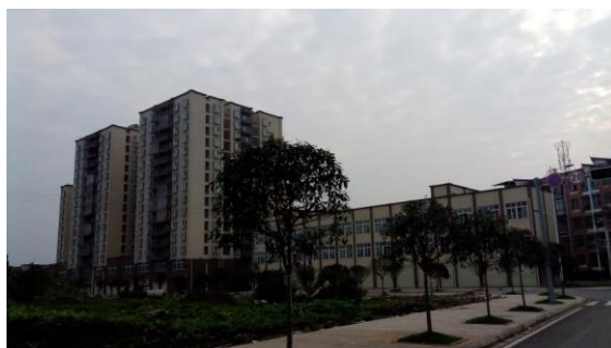
Figure 6-4 Completed Resettlement Houses in Mingshan District
