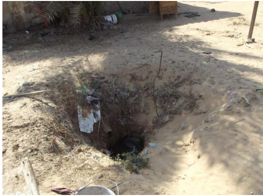
Figure 5B.20 The cesspit of El-Fukhary Landfill guard house
