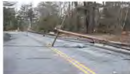
wind storm damage.
