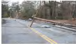
wind storm damage.
