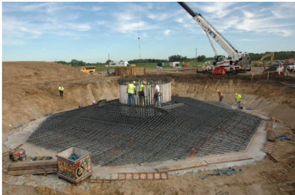
Figure 3.10 A Typical Turbine Foundation being Constructed
