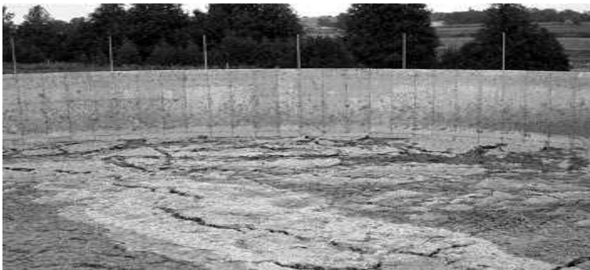
Figure 5.3: Crust Formation on a Liquid Manure Storage
