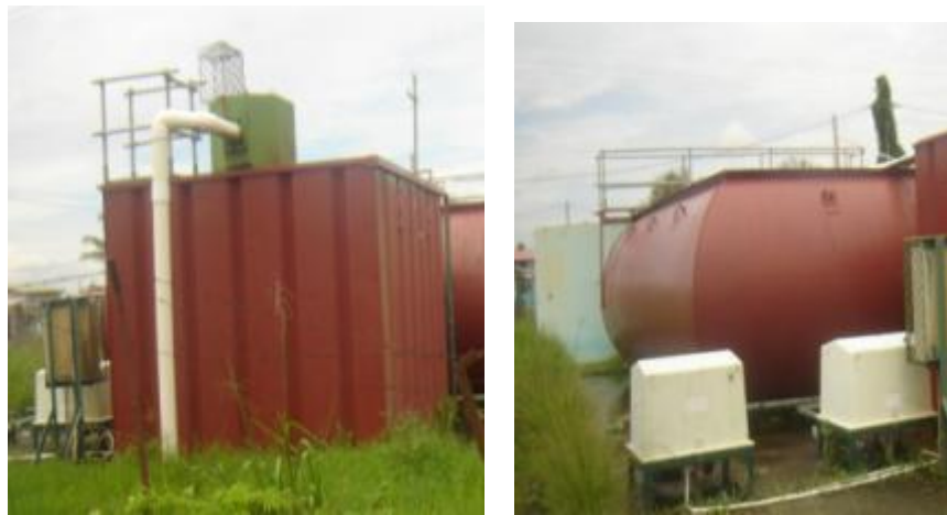
Primary Settling Tank and the Aeration Tank at the Turkeyen campus, University of Guyana. Source: Jackson, 2010b.
