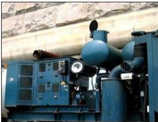
Figure 7.3.4.1.: Muffler system
