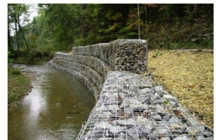
Gabion baskets for slope & river bank stabilization
