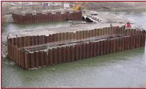
Figure 5.2: Steel sheet pile coffer dam for in-river construction activities
