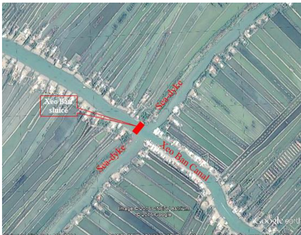
Figure 34: Location of Xeo Ban sluice
