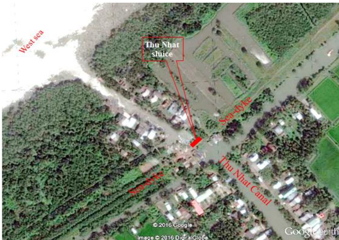
Figure 29: Location of Thu Nhat sluice
