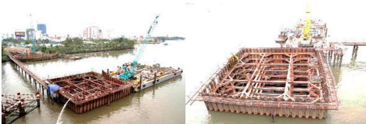
Figure 14: Construction of foundation pits by steel cofferdams
