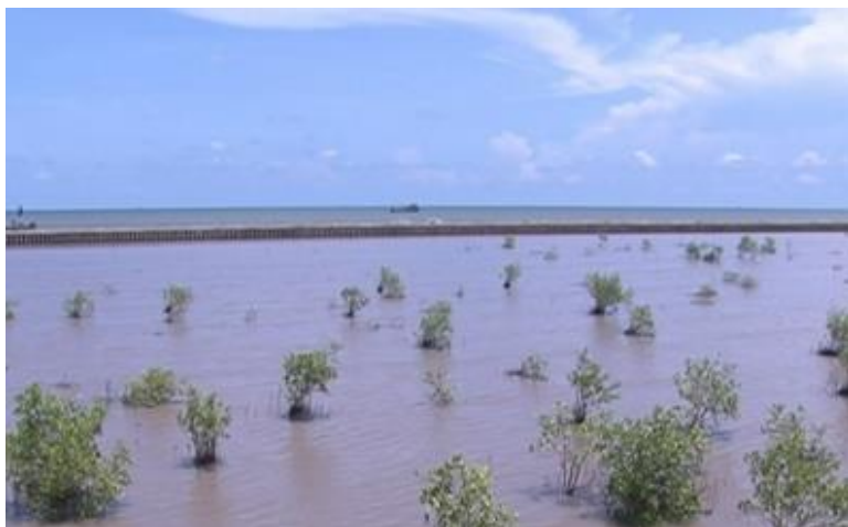
Figure 44: Under-water wave breaker for U Minh (Ca Mau) mangroves reforestation
