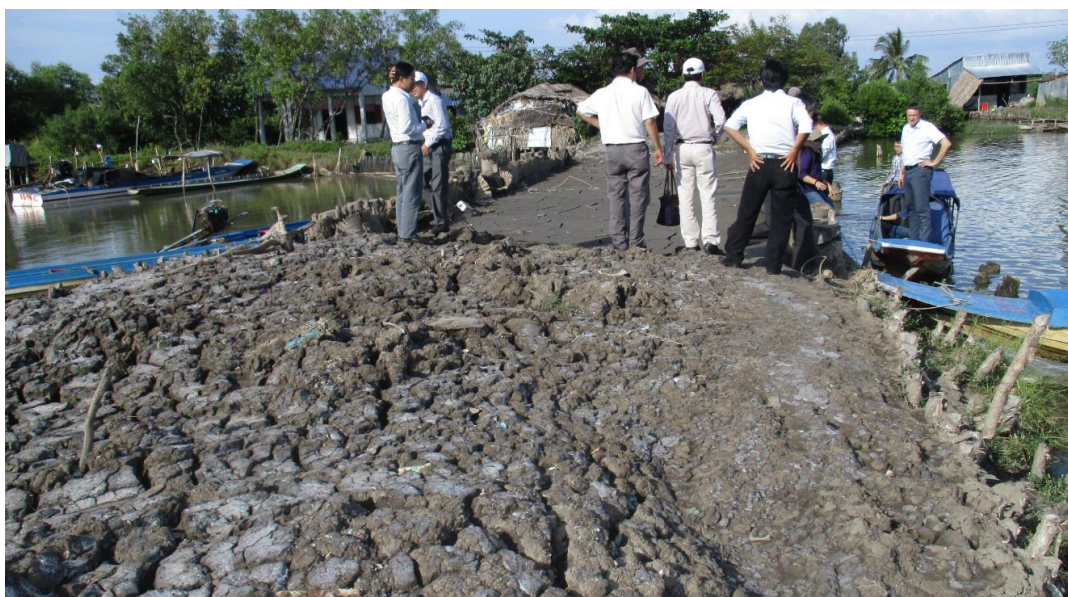
Figure 24: Temporary earth dam on Thu Chin canal
