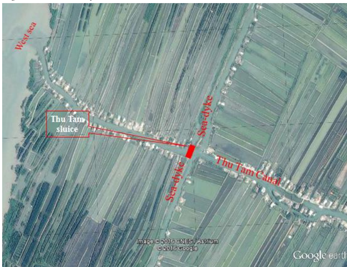
Figure 35: Location of Thu Tam sluice
