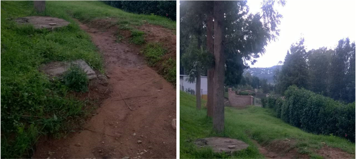
Plate 8: Septic tank and wall fence that will be affected by the development of R84 behind Maternity Ward
