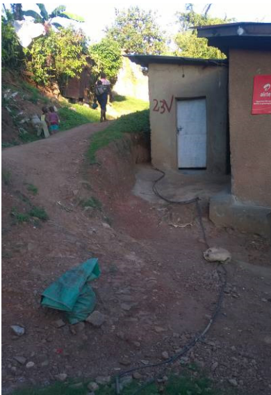
Plate 22: In Kiyovu Sector they are electrical cables and water pipes that are running above the ground crossing AS21, FP34 and AS22.
