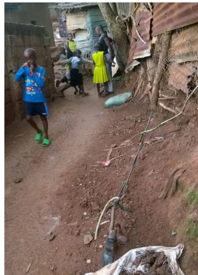
Plate 22: In Kiyovu Sector they are electrical cables and water pipes that are running above the ground crossing AS21, FP34 and AS22.
