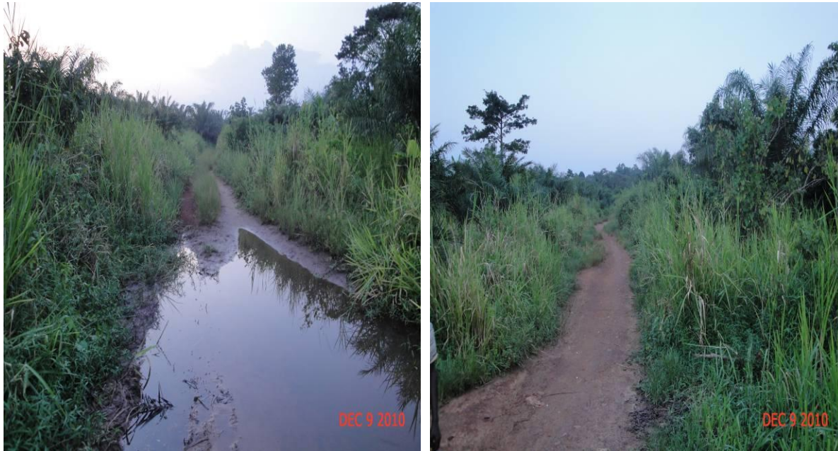
Figure 12.1 Sections of the Sampa- Ohuom Road covered by Weeds and Water
