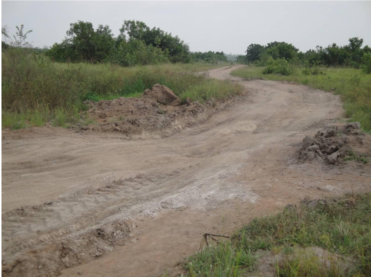
Figure 14.1 Typical Bad Section of the Akotsi-Gyinankoma-Ekroful Road
