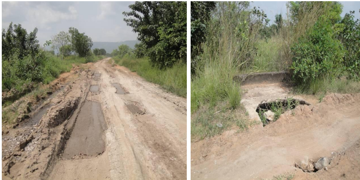
Figure 5.1 Portion of the Ayikuma Kordiba Roads and a Section showing Broken Culvert
