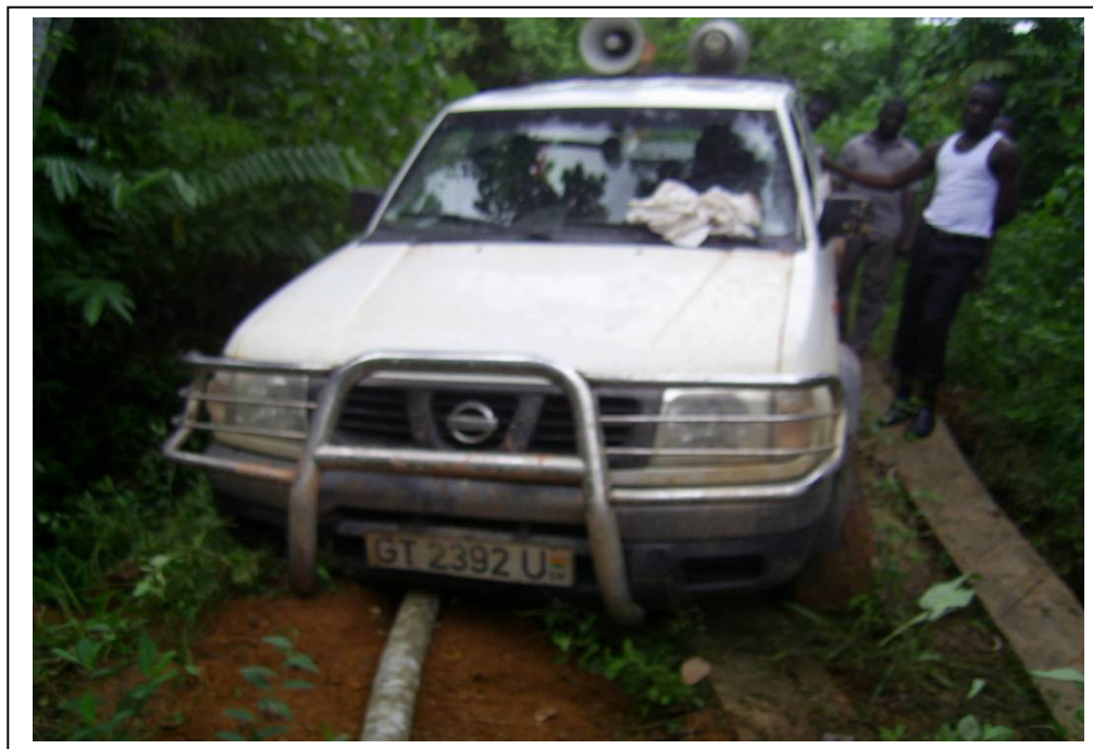
Figure 8.1 A car stuck on a section of the Gyampere-Kwasikrom Road
