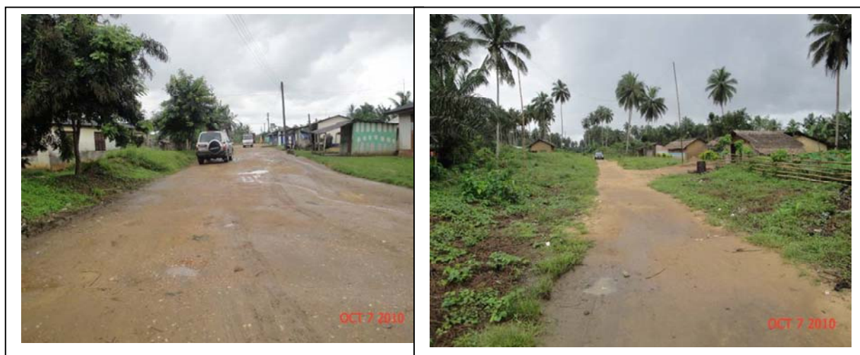
Figure 12.1 Sections of the Samenye-Etweakor Road in its current state
