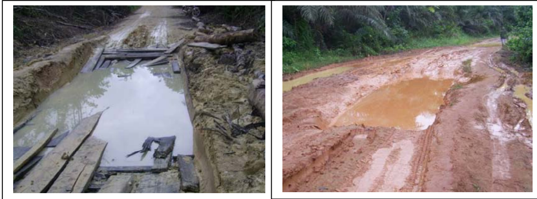
Figure 6.1 Some sections of the Domama-Adukrom Road
