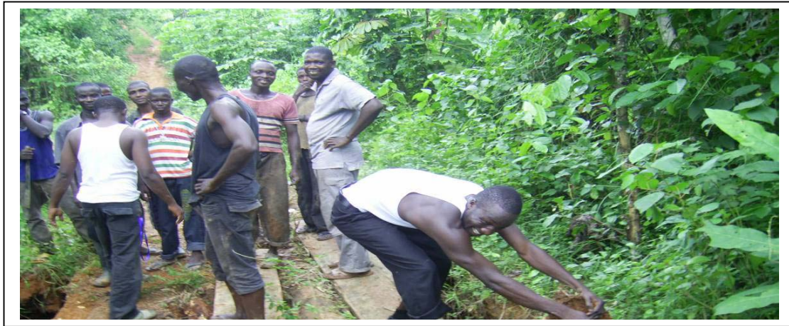
Figure 9.1 Community members improvising a culvert
