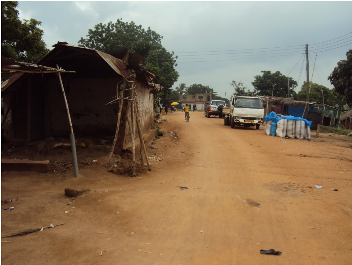
Figure 21.1 Sections of the Adawukwa – Ofadjato – Honi Road
