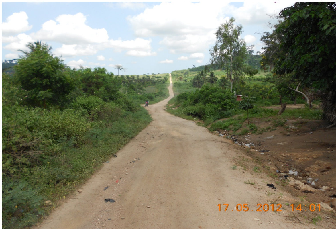
Figures 12.1a & 1b Sections of the Bewuenum – Adawukwa Road
