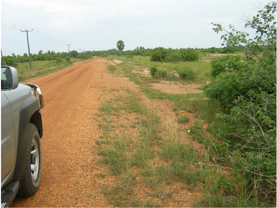
Figure 18.1 Sections of the Agortaga – Dalive Feeder Road
