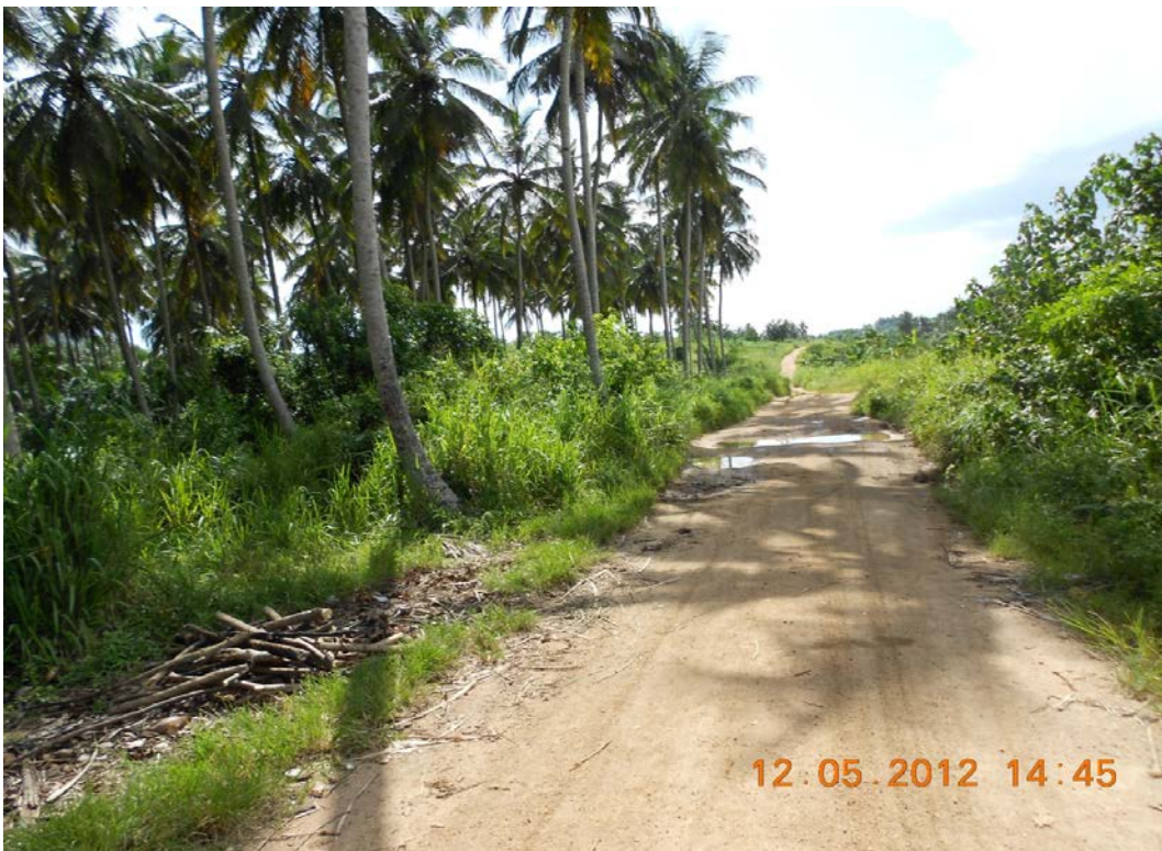
Figures 8.1 & 1b Sections of the Bawjiase – Aponkye Akura (Kwesi Adre) Feeder Road
