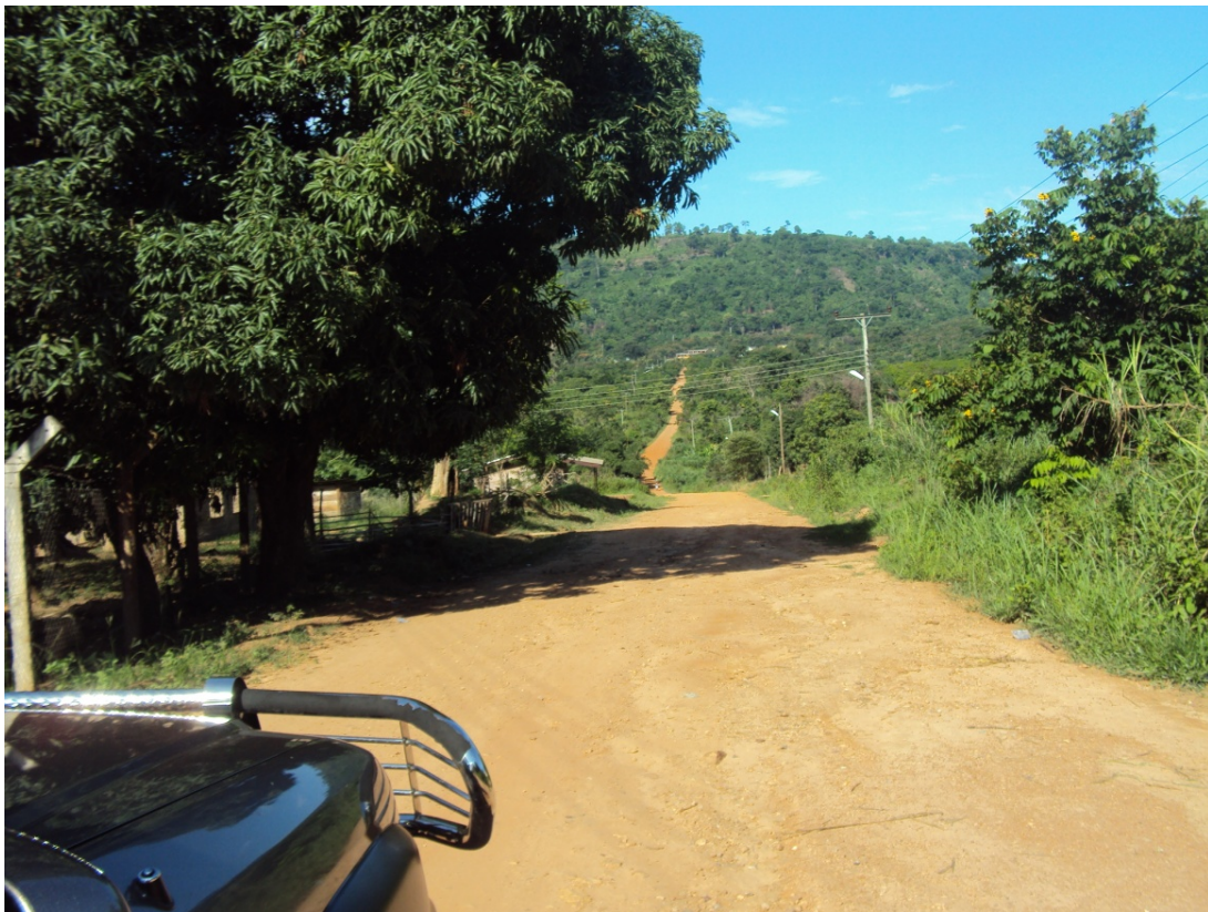
Figure 4.1 Section of the Nkonya – Gbi Wegbe Feeder. Road
