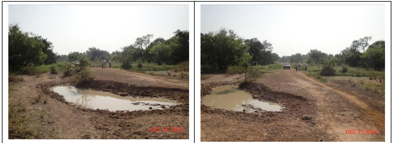
Figure 24.1 Typical Bad Sections of the Road
