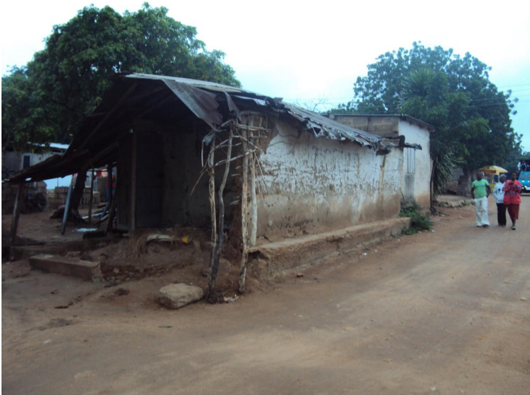
Structure on Adawukwa – Afadjato – Honi F/Rd
