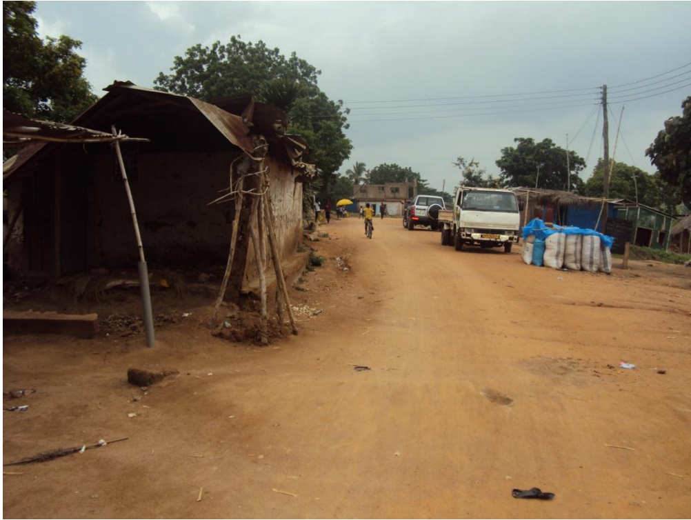
Structure on Adawukwa – Afadjato – Honi F/Rd
