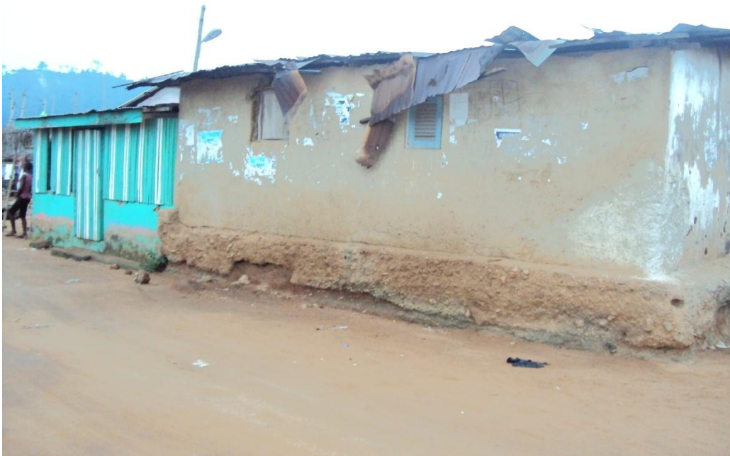
Structure on Adawukwa – Afadjato – Honi F/Rd
