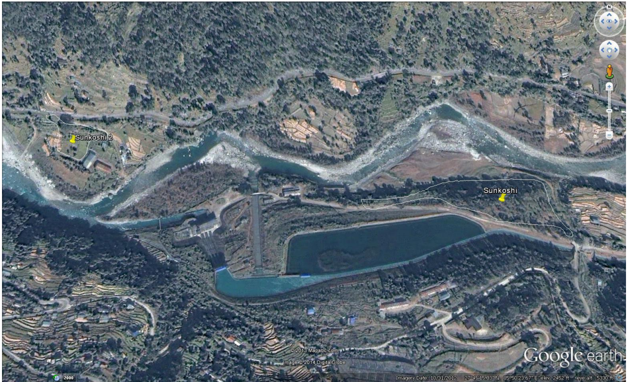
Figure 8: Sunkoshi 1 and 2 Sunkoshi Powerhouse Sites
