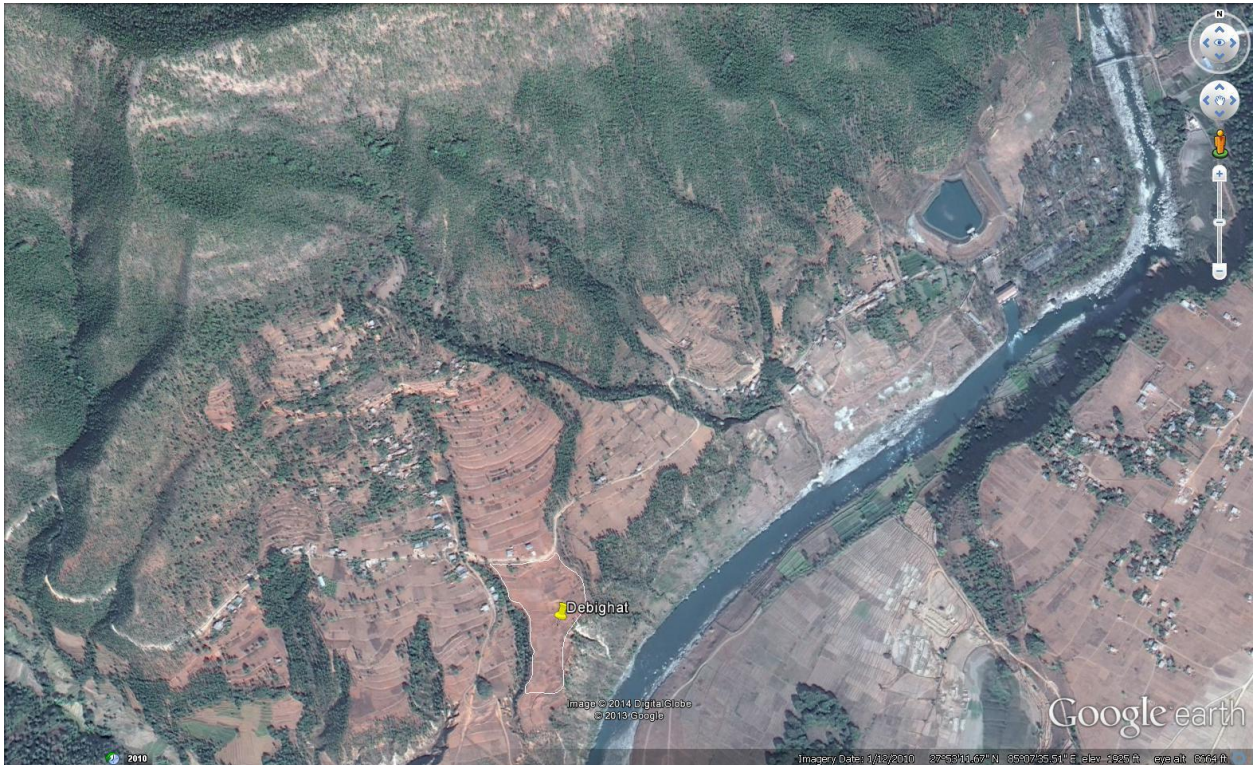
Figure 5: Devighat Powerhouse site
