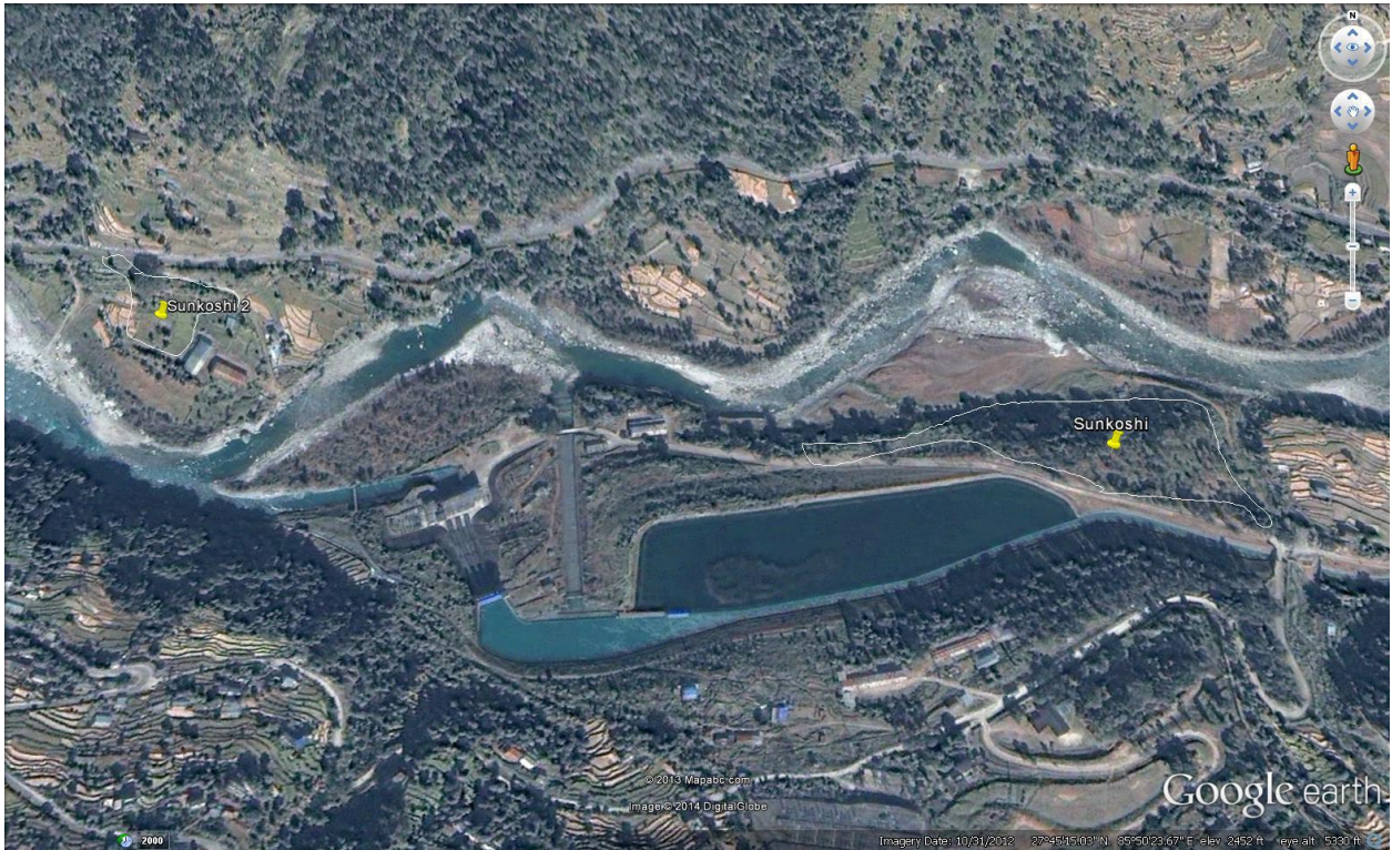
Figure 8: Sunkoshi 1 and 2 Sunkoshi Powerhouse Sites
