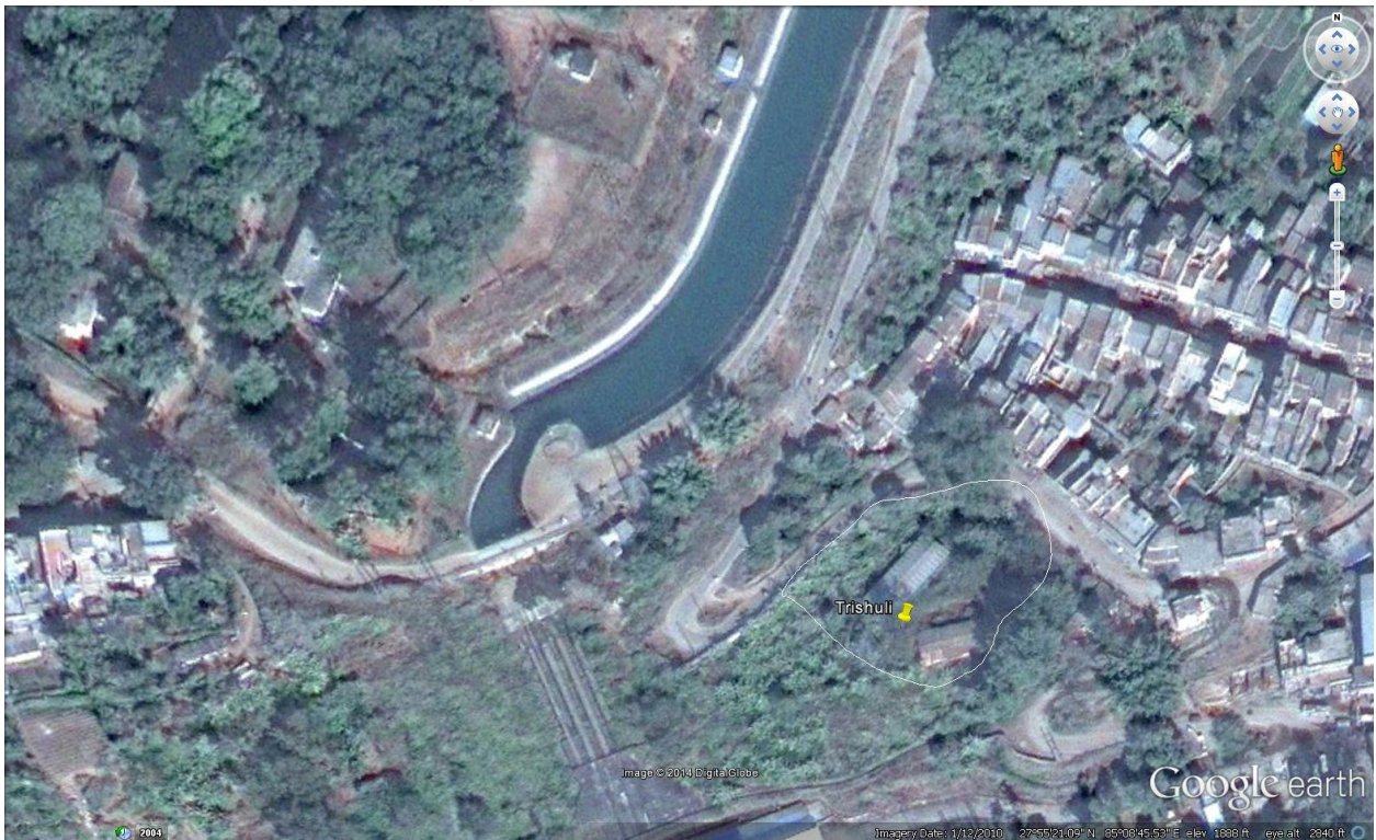
Figure 9: Trishuli Powerhouse Site
