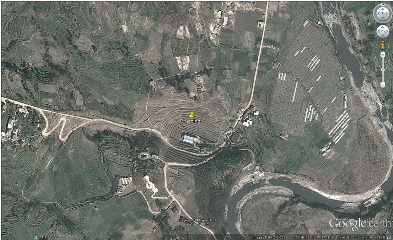
Figure 2: Pharping Powerhouse site
