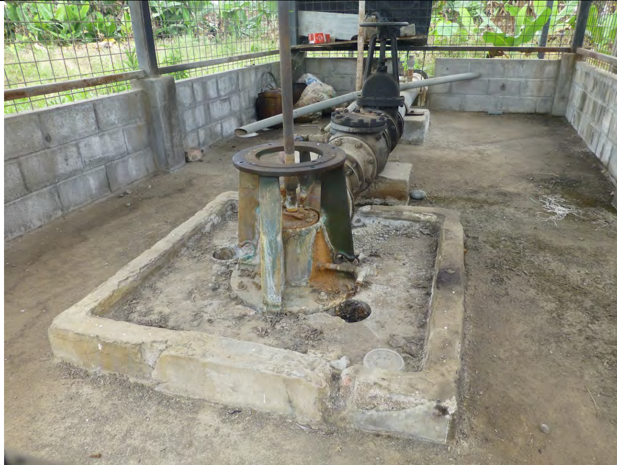
Well within a fenced and locked enclosure, deisel pump had been removed, casing not accesible.
