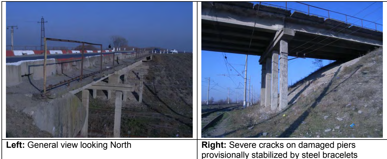
Figure 2: Photographs of Bridge No. 1
