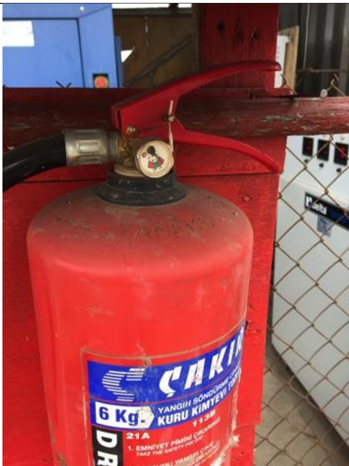
Fire extinguisher with low pressure in the construction camp.
