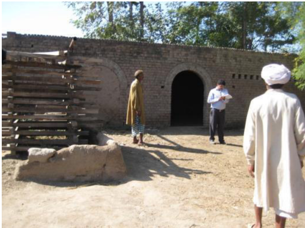
An Affected Structure
