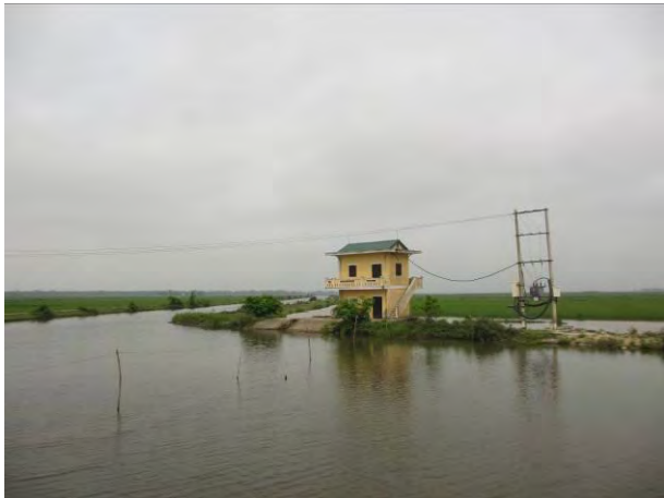
Photo 3: Water quality monitoring location at Hoi Tom Bridge (ending section)
