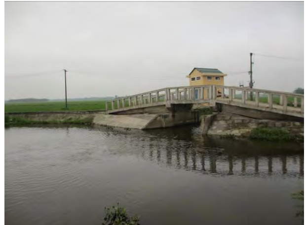
Photo 2: Water quality monitoring location at the beginning section (near Xa Ton pumping station)
