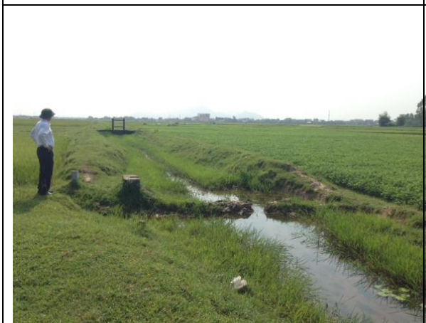
Upgrading on existing route
