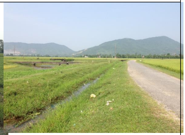
Upgrading on existing route
