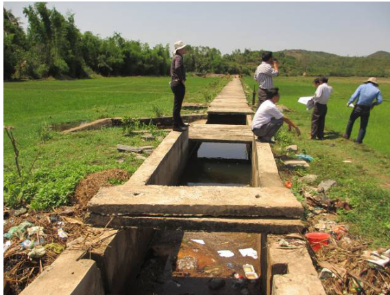
Photo 11: The main canal with rubbish
