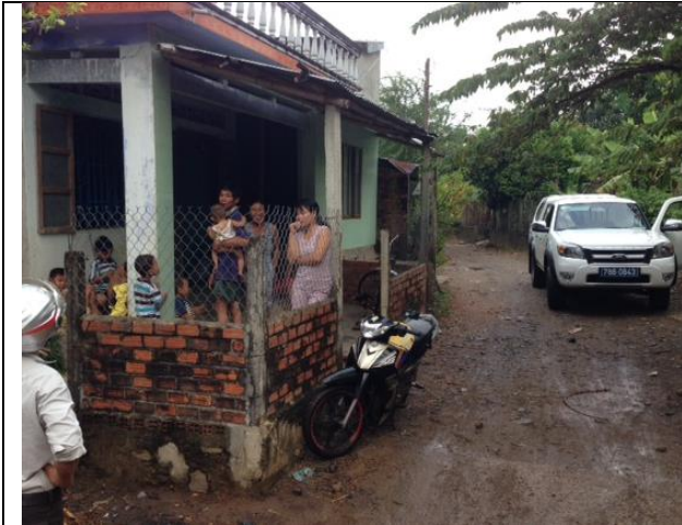
Affected fence by expanding road
