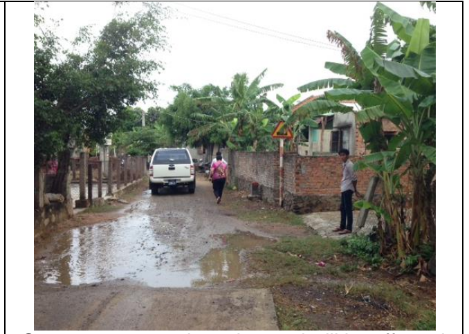
Some structures along the road will be affected
