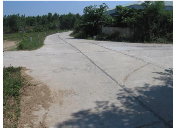
Photo 6: Public Safety monitoring point at Crossroad of Canal N3 management road ( Km 4+00) and commune road
