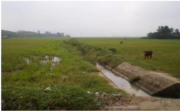
Photo 3: Branch canal N8-2 is eroded and canal bed is silted
