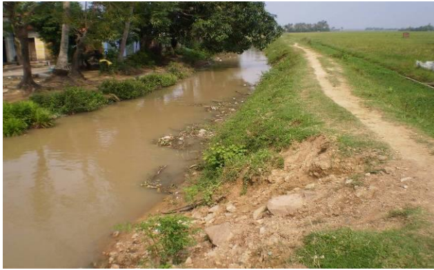
Photo 1: Existing status of Canal N3, taking water from North main canal & management road
