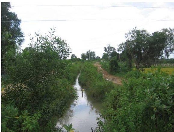
Photo 5: Existing status of primary canal N25
