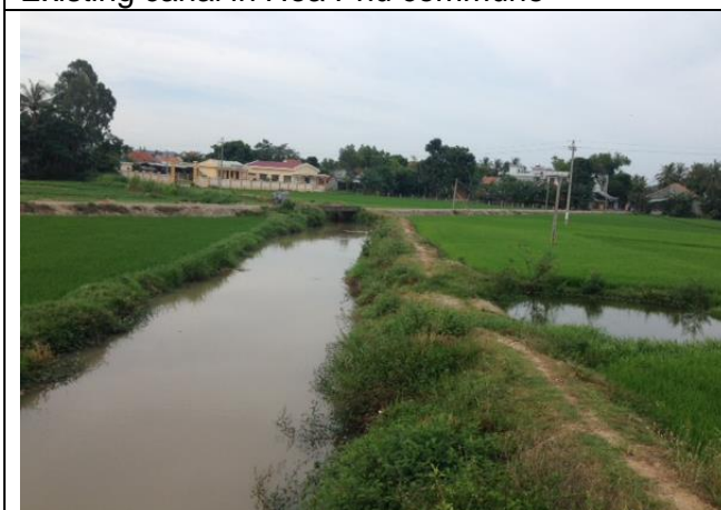
Existing canal and road in Hoa Kien commune
