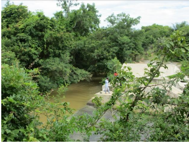
Photo7: Water quality monitoring point at the beginning section of northern main canal (at K0+500)
