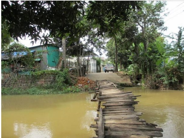
Photo9: Water quality monitoring point at K2+900 - northern main canal in Luong Cang 2 hamlet, Nhon Son commune
