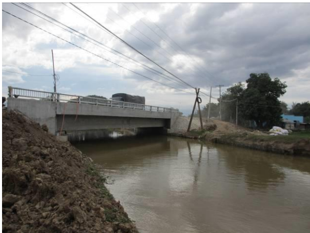
Photo11: Water quality monitoring point at Ong Mot bridge
