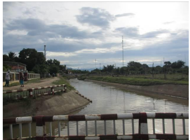
Photo12: Water quality monitoring point at regulator G2 (at K10+00)
