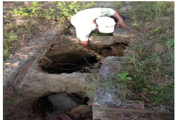
Photo 2: Eroded holes in downstream of Du Du Dam with depth >1m
