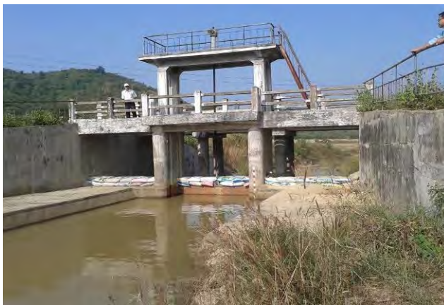
Photo 3: Spillway still good working
